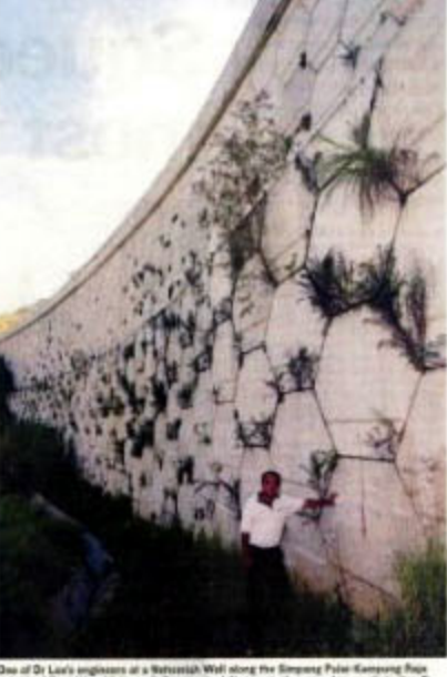
One of Dr Lee's engineers at a Nehemiah Wall along the Simpang Petai-Kemping Road stretch of East-West Highway E. Despite the hefty terrain that posed many obstacles, Dr Lee is proud to say that his company built the country's highest reinforced soil wall.
